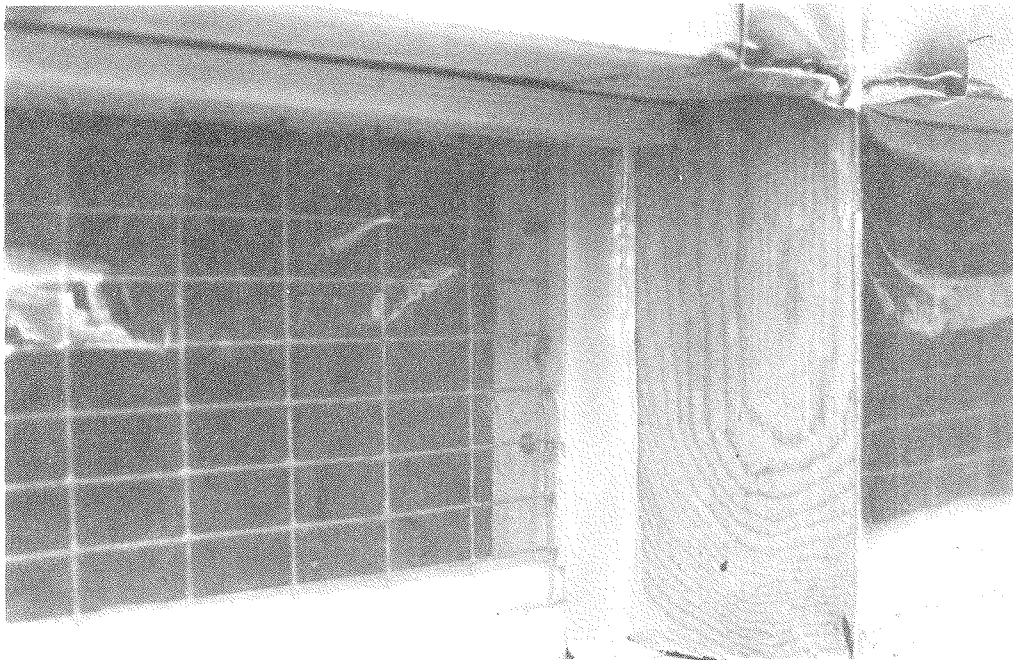
Figure 2.20 Top damper of the internally ventilated Trombe wall. Note the grid and the Teflon foil.
