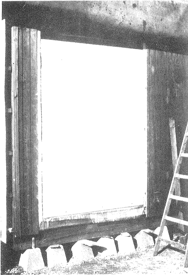
Figure 2.4 The mass component before installation of the rest of the solar wall.
