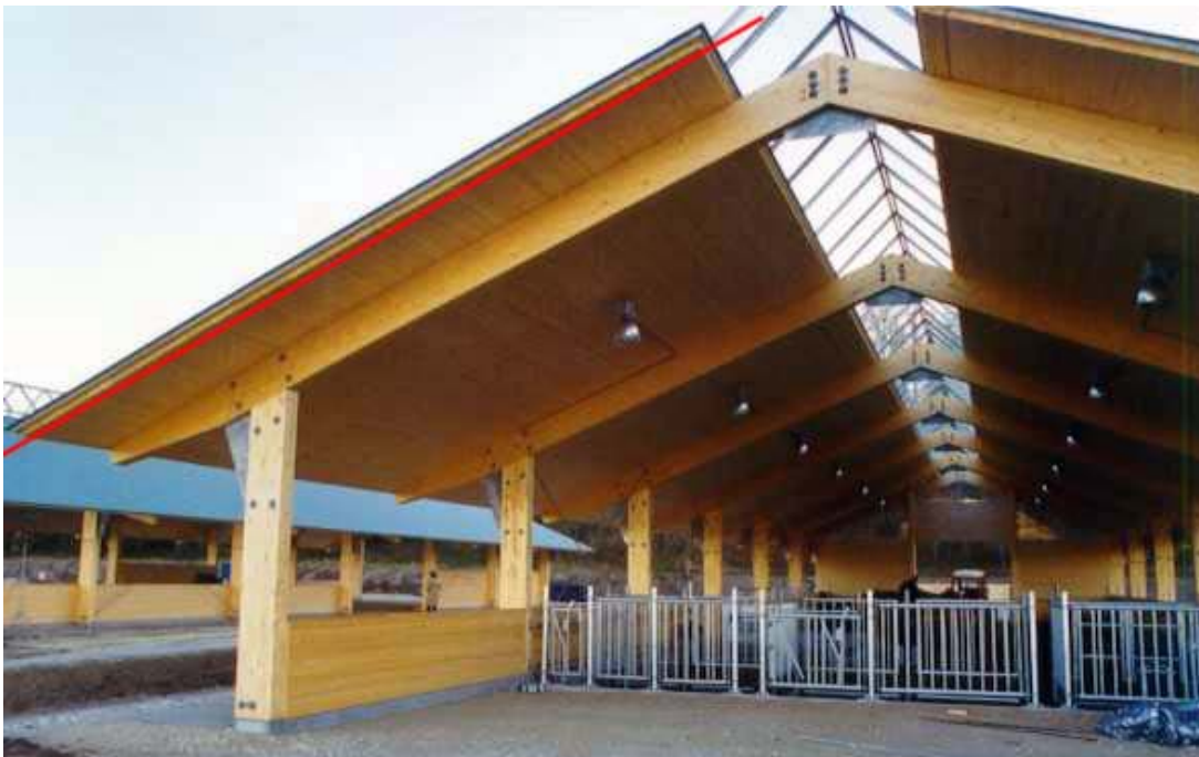
Figure 1: Glued solidwood elements used as roof elements at outdoor covered climate conditions – a slight rise of the otherwise straight roof plane is observed, the rise is probably a function of restricted moisture swelling of the individual elements.
