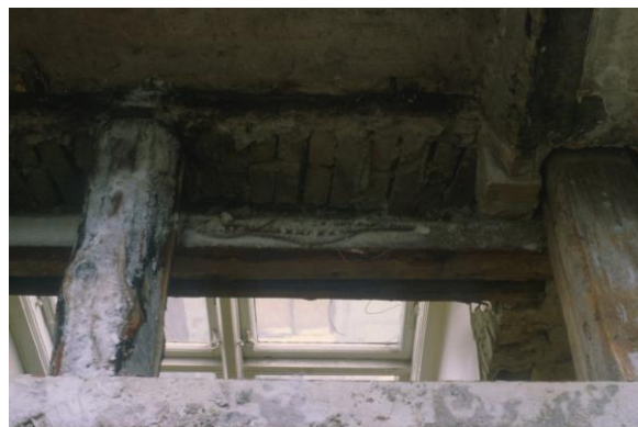
Fig. 2: Support of beams in the wall (danskbyggeskik.dk).
