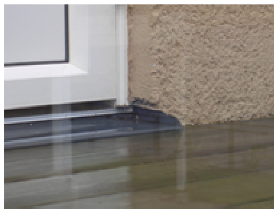
FIG 11. A poor connection to a patio door.
