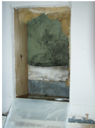
FIG 3. Microbial growth on the outer gypsum board, caused by water leaking in through a defective connection. Picture from the inside.
