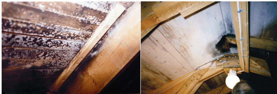
FIG. 1: Example of moisture damaged attics.
