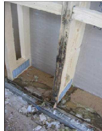
FIG 4. Microbial growth on sole plate and studs, caused by inward leakage of water. Picture from the outside.
