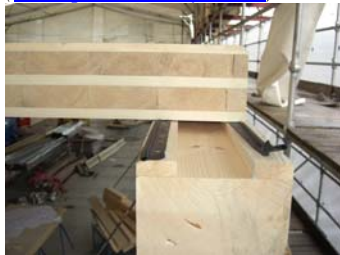
Fig. 3 Examples of mounting of massive timber elements, roof on walls.
