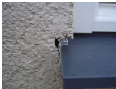
FIG 12. A poor connection around a window
