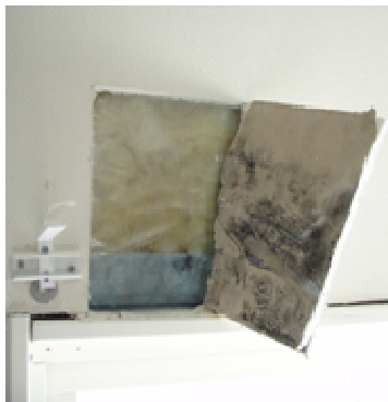
FIG 2. Microbial growth on the internal gypsum board, caused by inward-leaking water.
