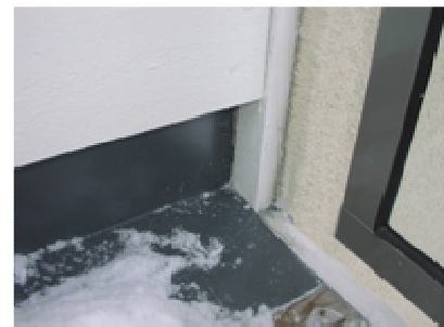
FIG 13. Leaks around the edge of a balcony.
