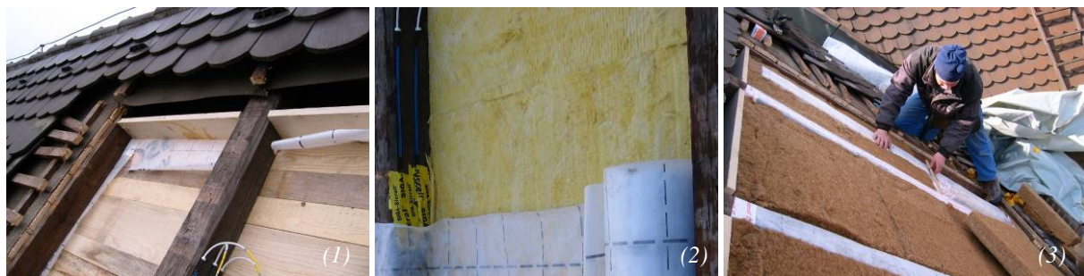
Fig. 3: Variation 2 under construction – open roof with boarding (1), vapour barrier over rafters (2), installation of hemp insulation (3)
