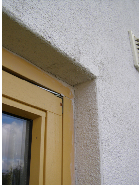
FIG. 5: Example of insufficient tightening around windows in a one-stage tightening wall construction of aerated concrete blocks. The plastering is the only rain- and wind barrier around the openings.
