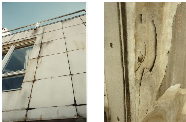
FIG. 10: Example of construction with cement based sheets. Due to insufficient ventilation and drainage of moisture the sheets were damaged by frost.
