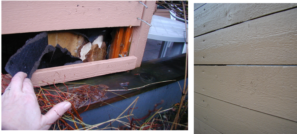
FIG. 999: Example of a construction with openings in the façade and limited drainage openings.
