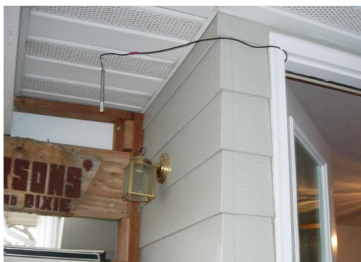
FIG. 7: Location of exterior climate sensor
