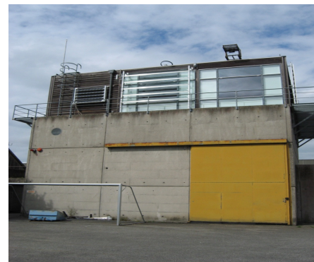
FIG. 6: Picture of the glass lamella system mounted on the test room façade.
