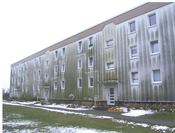
FIG. 1: Compact algal growth on the northern facade of a thermally upgraded building
