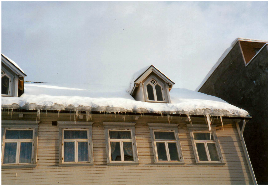
FIG. 5: An old house with icicles at the gutter filled with ice (photo Anker Nielsen)
