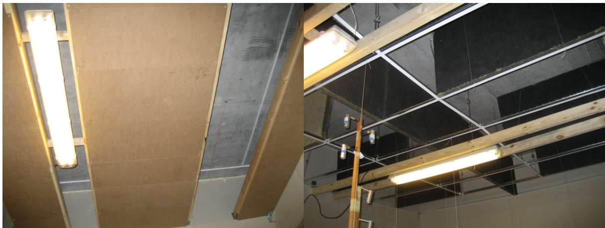
FIG. 4: Pictures of acoustic ceilings – left a plywood lowered ceiling and right acoustic panels as baffles
