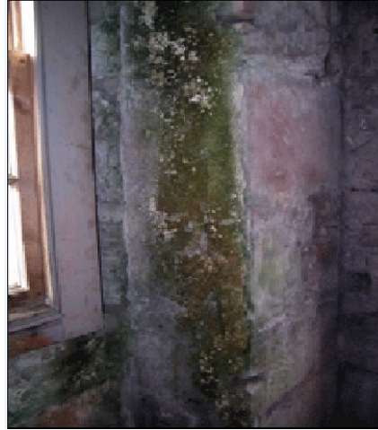
FIG. 1: Moisture damage to interior of the castle
