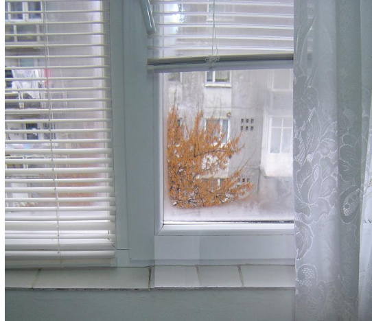
FIG. 1: Window having a PVC framework placed in a wall made of big prefabricated panel of 27 cm thickness with condense on the interior surface of the glass
