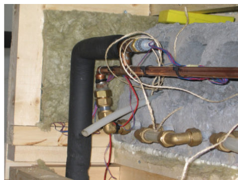
FIG. 1: View of the hollow core concrete deck in which the TABS is integrated
