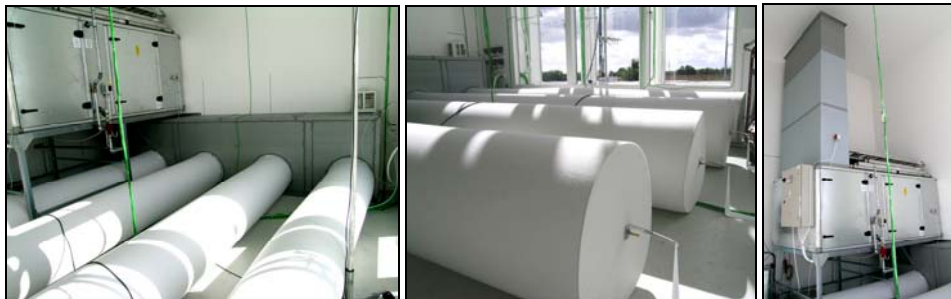
Figure 3. KE-low impulse fabric ducts in the experiment room (left, centre), Ventilation system in the experiment room (right).
