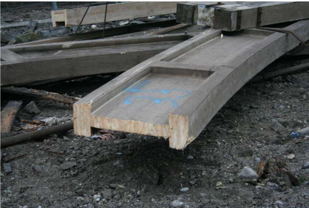
Cross section in glulam arch
