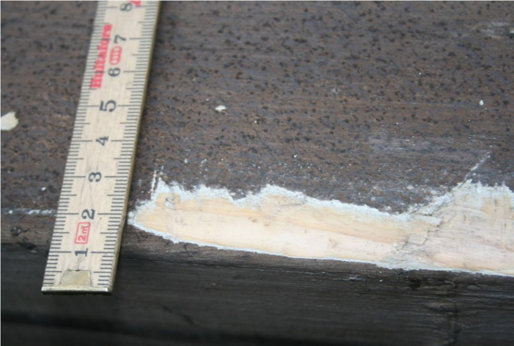
Scarf joint. The surface coating has been cut away to show that the scarf joint is OK. No delamination.
