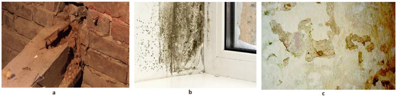
Figure 9: a) decayed beam end, b) mould around window, and c) mould on cold surface
