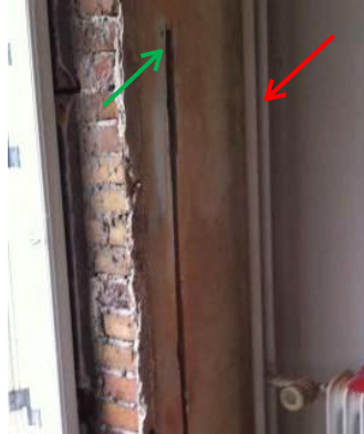
Figure 15: Hot water pipes (red arrow) in the vicinity of sensor 6 location (green arrow)
