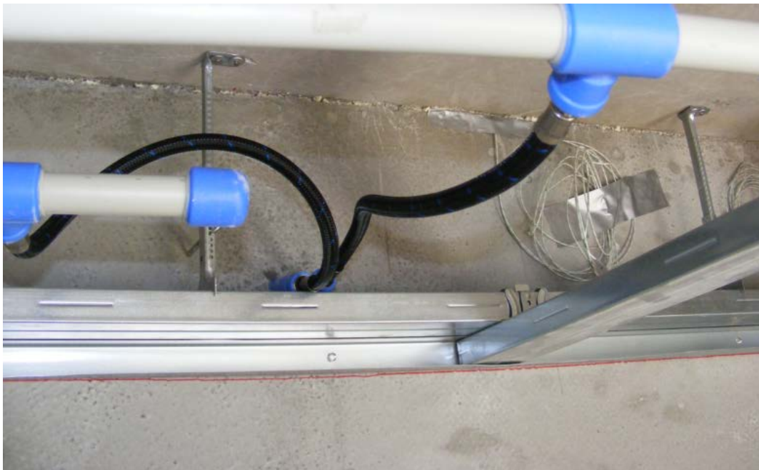
Figure 17: Connection of capillary mats with manifold pipes
