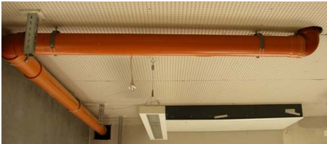
Figure 14: Drainage pipe situated below suspended ceiling
