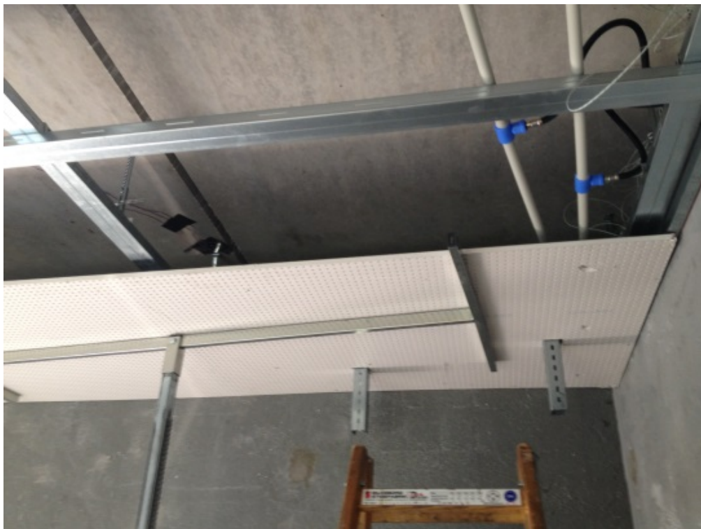
Figure 23: Installation of suspended ceiling
