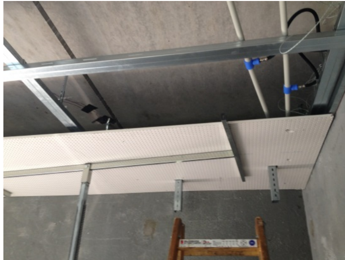
Figure 1: Diffuse ceiling inlet construction and connection of capillary mats to manifold pipes
