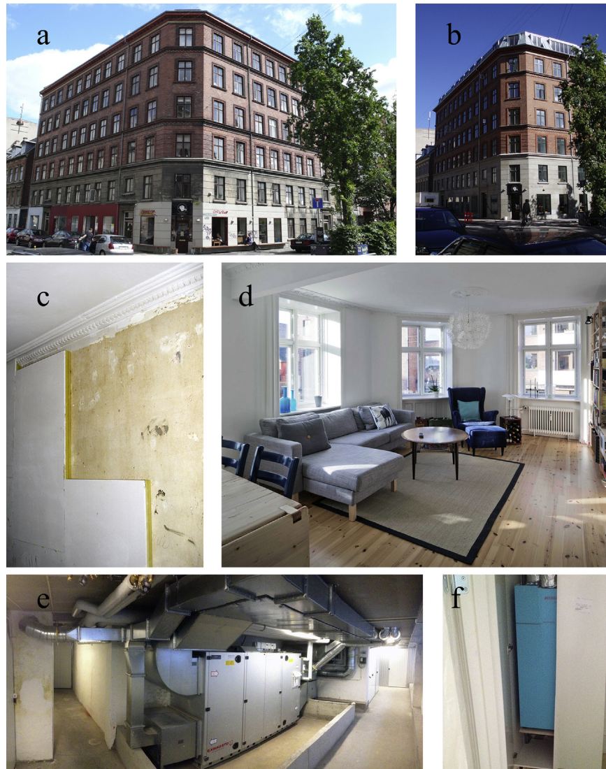
Fig. 1. a) The building before renovation. b) The building after the renovation. c) Internal insulation applied. d) New energy efficient windows with 3 layered glazing constructed aesthetically as the old once. e) AHU in basement for central ventilation systems in Block A and B. f) AHU for decentralised ventilation systems in Block C.
