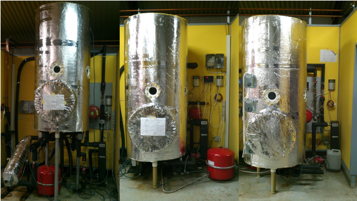
Figure 20. The heat storages of the three solar heating systems which are being tested.
