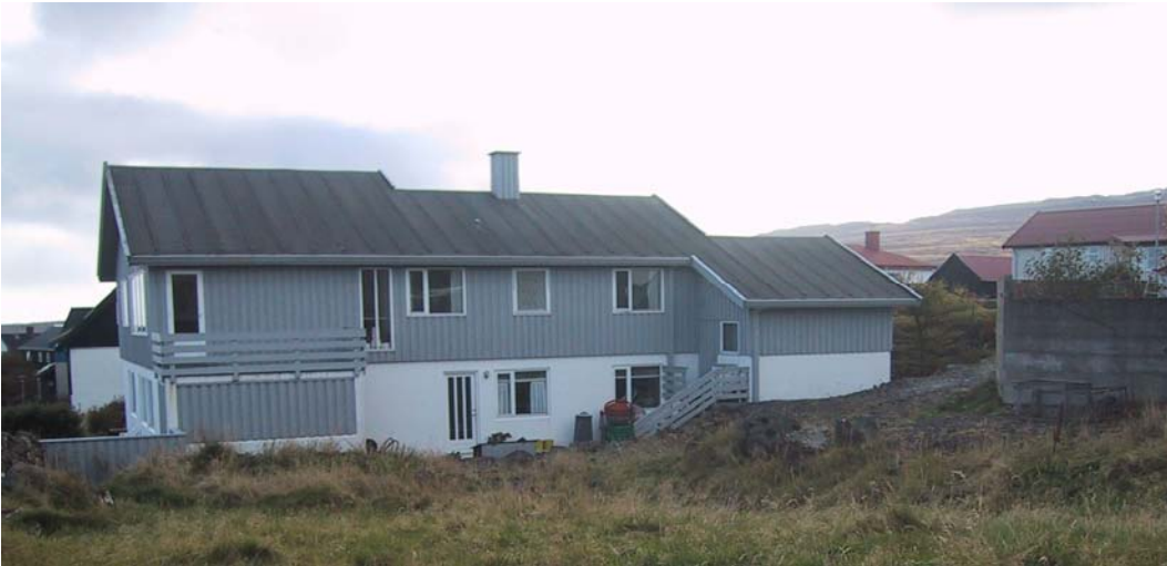
Figure 3 A typical Faroese single family house of a type that has been the dominating style since the 60'ies with full basement made of cement and the main living floor made of wood. It is common to expand the living area to the basement when the children want more space and privacy.
