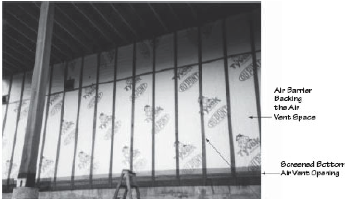
Figure 4: A photo of a ventilated exterior cladding system under construction in Southeast Alaska. (From an English translation of the NBI publication “Byggedetaljer: NBI Byggforsk A542.003”, also published as Alaska Building Research Series HCM-01558, with additions and used with permission, 1988)
