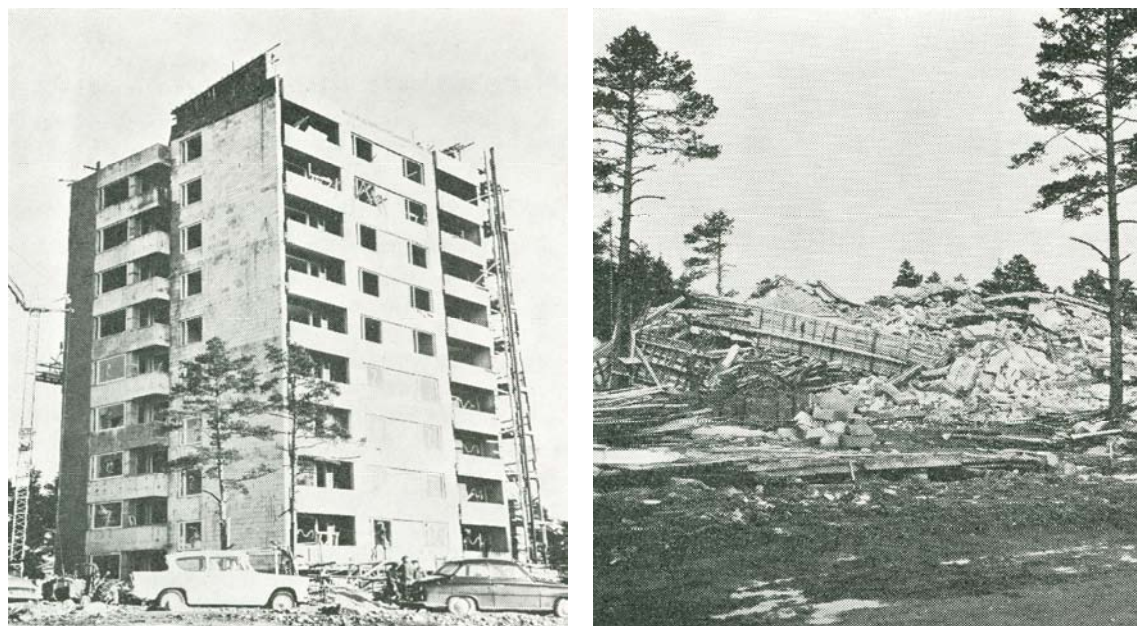
Figure 1 The collapse of a 9-story building due to premature freezing of the load-carrying concrete (Nykänen (1964)). This type of difficulties are easily prevented with simple precautions during the casting and early hardening.
