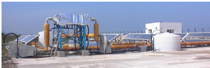
Fig.1.2: Photo of the one-stage pilot plant constructed, including a spray evaporation unit [7].
