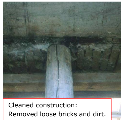
Figure 30 Cleaned up construction: Wooden beam supported by a wall plate in between masonry columns.
