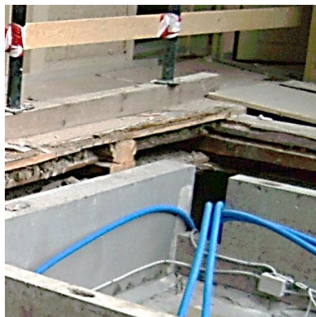
Figure 24 Wooden floor structure, note the recess in the wooden beam for pugging boards.
