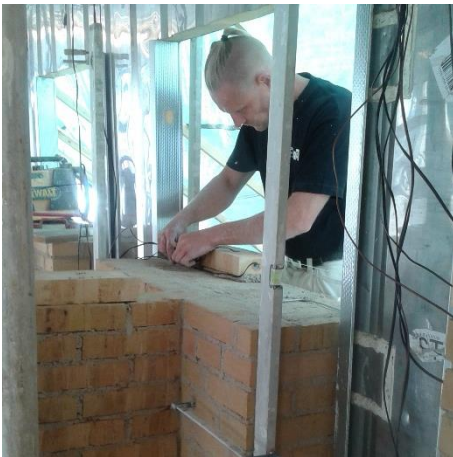
Figure 77 Mason installing brick with pre-installed sensors at measurement point 1.
