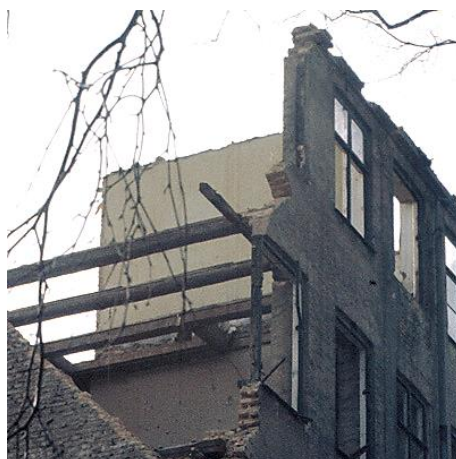
Figure 26 Wall plates and beams uncovered during demolition of building.
