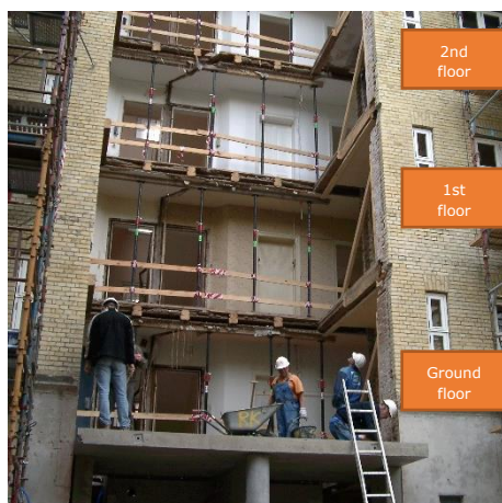
Figure 17 Opening of courtyard facade, photo showing ground until 3rd floor.
