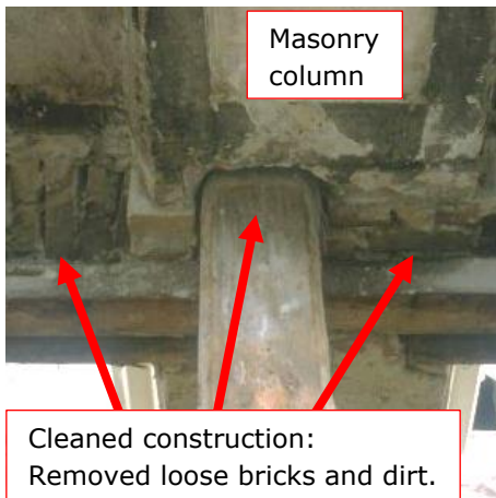
Figure 29 Cleaned up construction: Wooden beam end in masonry column, supported by a wall plate.
