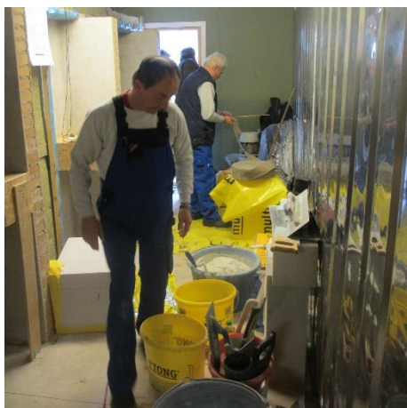
Figure 79 Thermal insulation is installed by the producers following system guidelines.
