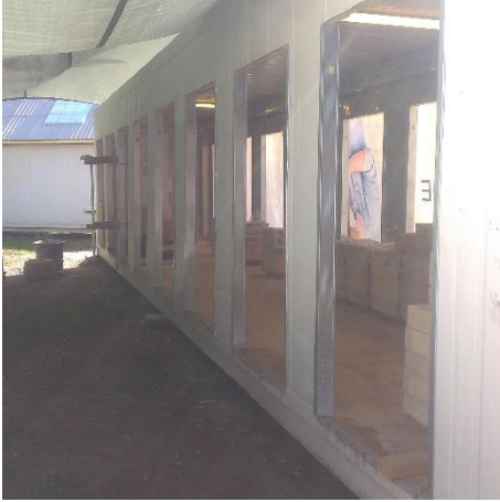
Figure 75 Perforated container C3.
