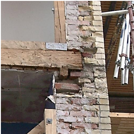
Figure 21 Facade/wooden beam interaction, 2nd floor (2 bricks) --> 3rd floor (1½ bricks).
