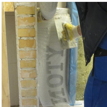
Figure 80 Thermal insulation is installed by the producers following system guidelines.
