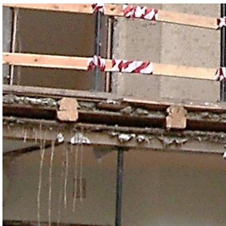
Figure 23 Wooden floor structure with wooden beam and pugging layer.
