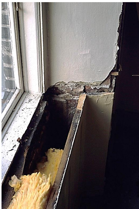
Figure 33 Timber finishing in front of spandrel. In some cases retrofitted with thermal insulation.
