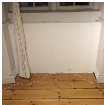
Figure 123 Interior surface of insulated spandrel in room 09.
