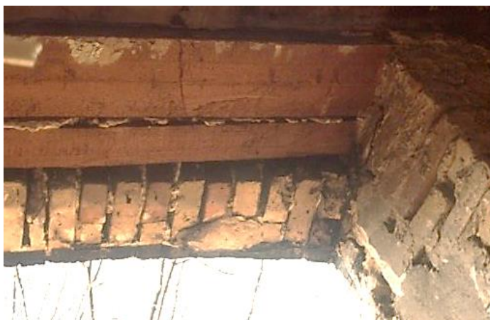
Figure 35 Lintel over window in façade. Photo courtesy of J. Engelmark
