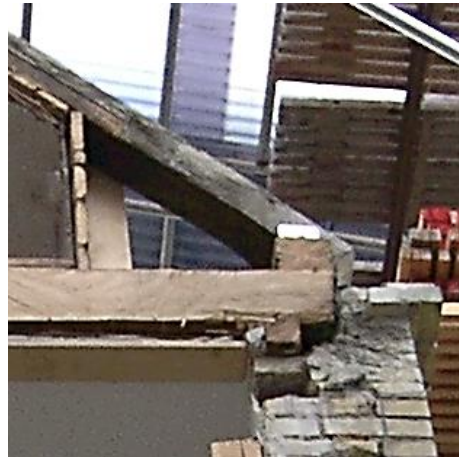
Figure 22 Facade/wooden beam interaction, 3rd floor (1½ bricks) --> 4th floor (roof).
