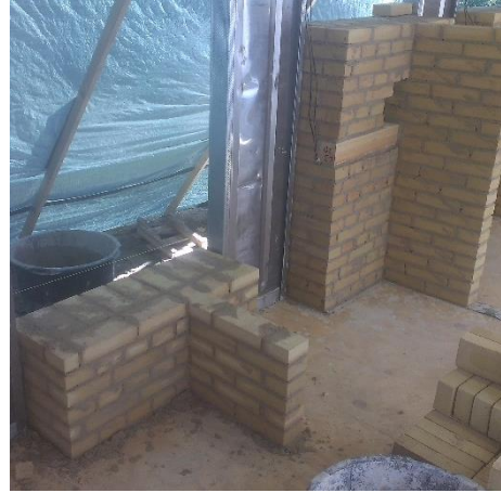
Figure 76 Construction of solid masonry walls with embedded wooden elements.
