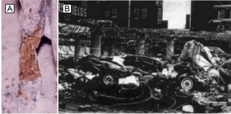
Figure 5.18: [A]: Notch-like shape corrosion attack of rebar in chloride contaminated concrete. From [COWI, 2007b]. [B]: Collapse of parking garage in Minnesota, USA, due to chloride induced corrosion damage. From [Borgard et al., 1990].
