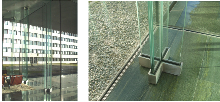
Figure 1.3: Load bearing glass columns at the headquarters of Danfoss, Denmark, by Schmidt, Hammer & Lassen. Each column carries a vertical load of 250kN . Photo: Rambøll.
