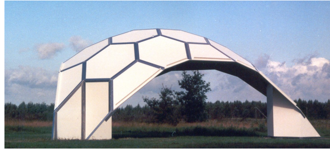
Figure 1.7: Full scale model of plate shell structure in 19mm plywood, located at the Danish Building Research Institute, Denmark. Designed by Henrik Almegaard. Illustration from [9].
