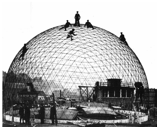
Figure 2.4: Construction of the Zeiss Planetarium in Jena, Germany, designed by Walther Bauersfeld in 1923 [29].
