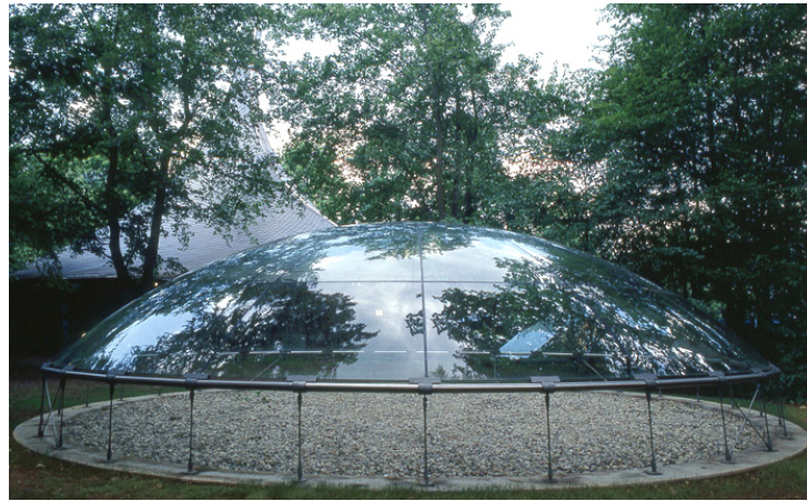
Figure 1.4: Glass dome at ILEK [16]. The glass segments are doubly curved laminated glass with a total thickness of 10mm , connected by glued butt joints with a width of 10mm . The diameter of the shell structure is 8.5m . Photo: ILEK.
