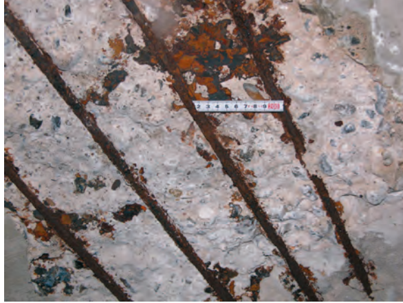
Figure 2.3 Typical example of a severe general corrosion attack in uncarbonated concrete, caused by excessive amounts of chloride.
