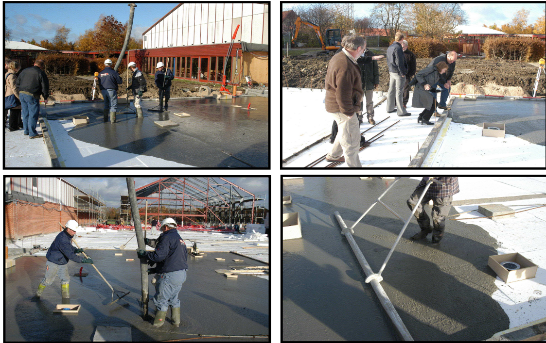
Figure 2.1 An example of a simple horizontal SCC application, in this case an in-situ floor. Drainpipes are typically used to level the surface (Wallin 2003).
