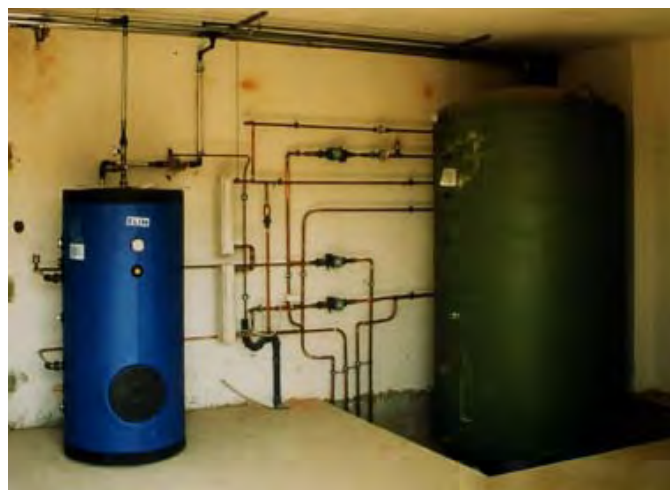
Fig. 2–3 Solar combisystem with extra domestic hot water tank.
