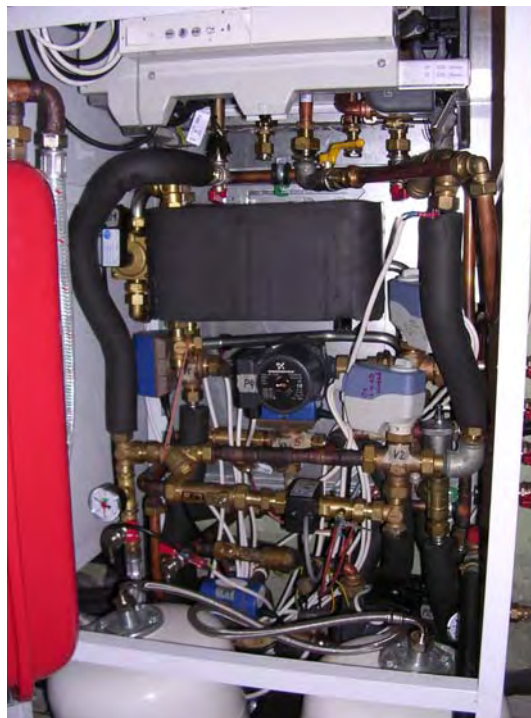
Fig. 6–11 Hydraulic unit inside the technical cabinet in the demonstration system; the big black box is the insulated domestic hot water heat exchanger, below the main pump P4 can be seen.
