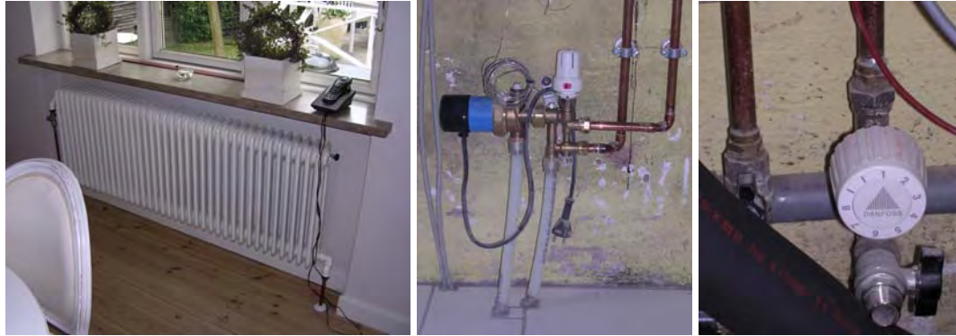
Fig. 6–2 Cast iron radiator in the dining room (left), the pump with integrated mixing valve for the bedroom in the basement (middle) and the return flow control thermostat valve for the floor heating in the bathroom in the basement (right).
