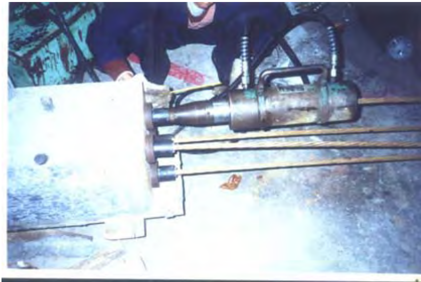
Fig.2.3 The process of tensioning and grouting
