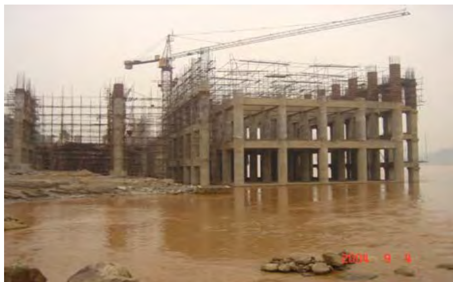
Fig. 5.4 Hydraulic structure of container berth
