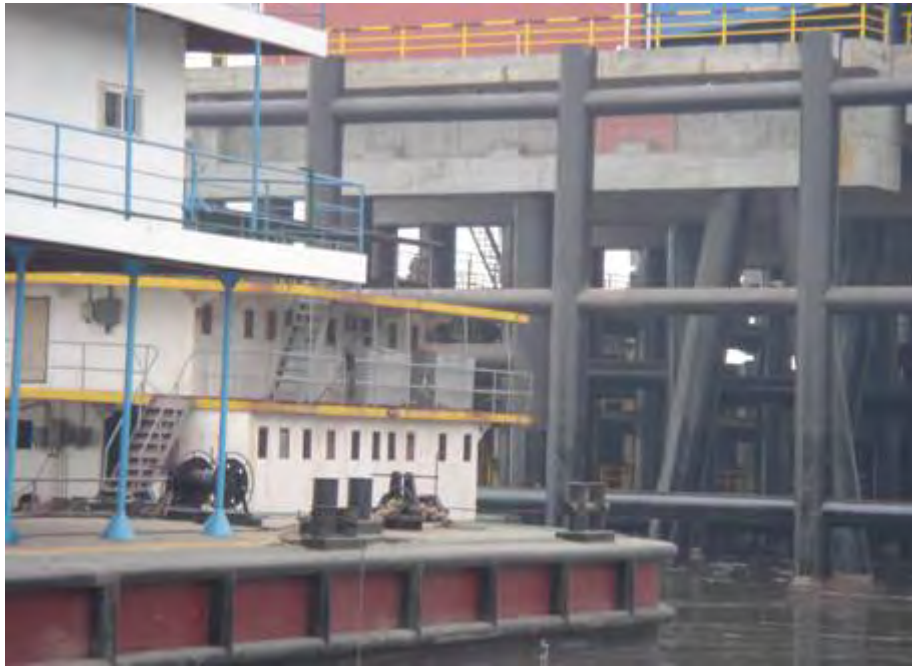
Fig.1.7 Steel berthing pile
