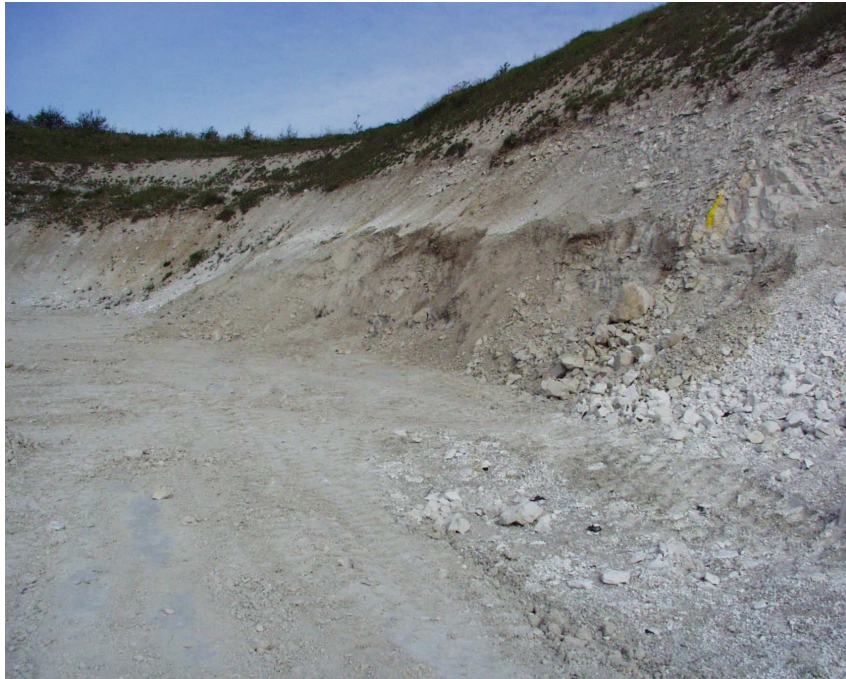
Figure C.4 Excavated chalk wall (approximately 2.5 m high and 25 m long).
