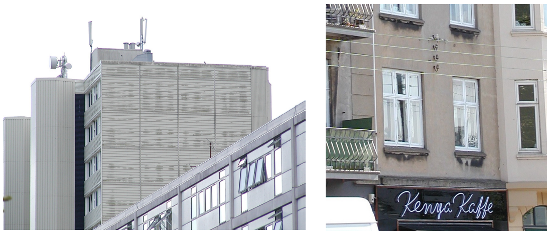
Figure 3.6: Soiling patterns indicate the origin of the dirt. Left: biological growth at exposed moist areas. Right: in polluted areas the rain will wash off some of the particles in unprotected areas. The rain will not clean areas under protective items like sills or coverings. This results in darker areas under protective items.
