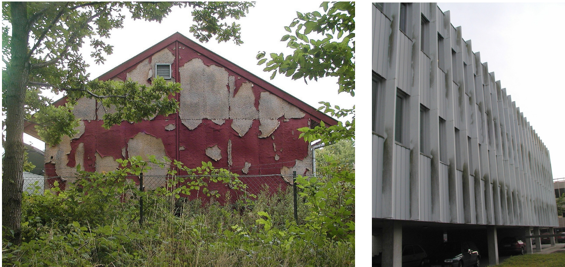
Figure 4.7: Different surface failures. Left: the surface paint is not intact and the underlying material is no longer protected. Right: algae growth at a white aluminium facade. Although the facade is still protected, the surface has failed because the building looks dirty and is in contrast to the image the building owner wants.
