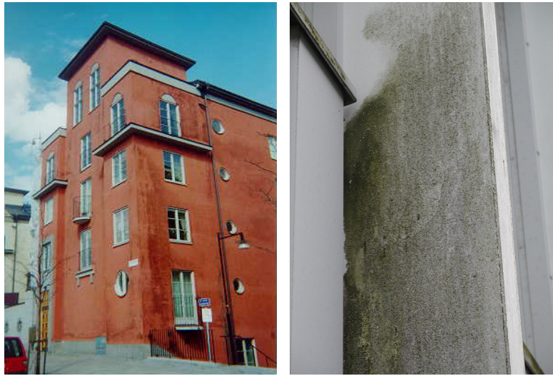
Figure 4.10: Examples of unacceptable soiling. Left: mould growth at a two year old house. Right: Algae growth at aluminium facade, three years after cleaning with brush and water. Both buildings had to be cleaned, despite the risk of higher susceptibility to soiling.
