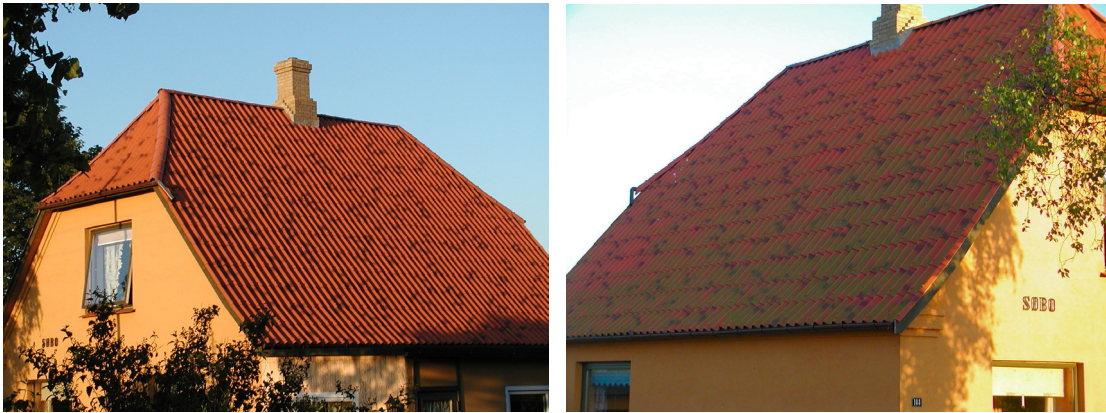
Figure 3.2: Eternite (fibre cement) roof fabricated with “pre-soiling” patterns. The patterns give the surface more life but are different from the natural soiling pattern. At the northern side of the roof (to the right) algae growth has resulted in a greenish discolouration of the roof.
