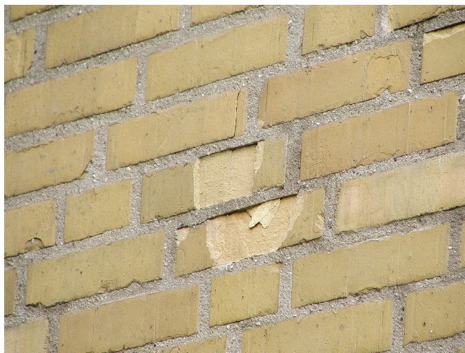
Figure 4.1: Scaling of bricks due to frost damage. Some of the bricks in this detached wall are not frost resistant; 0.5 cm thick layers scale off the brick.
