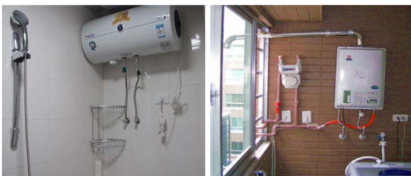
(a) Storage-type electric water heaters (b) Natural gas water heaters
