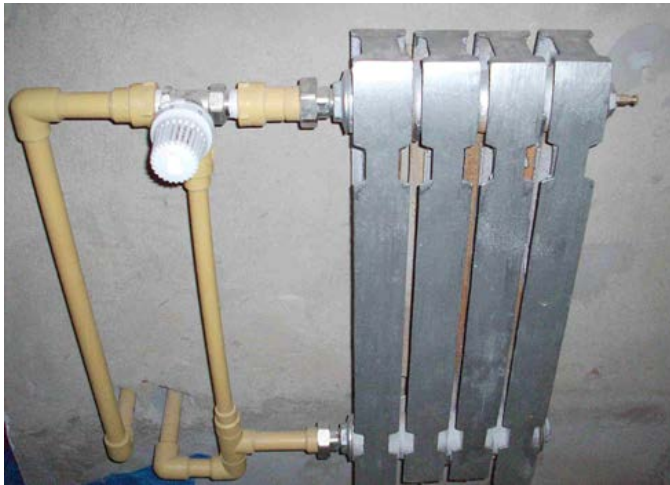
(a) Old radiators equipped with TRV in China
