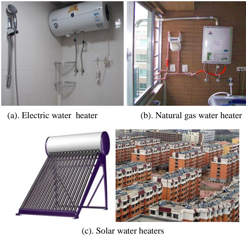
Figure 2. Individual water heater installations in Chinese households
