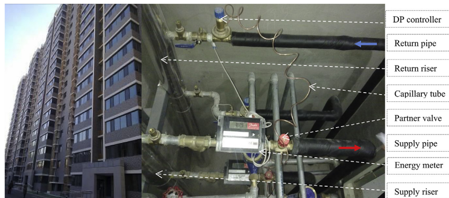
Fig. 7. Real test case for the flow control approach.
