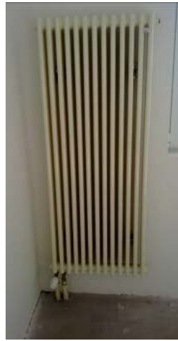
(b) New radiators equipped with TRV in China
