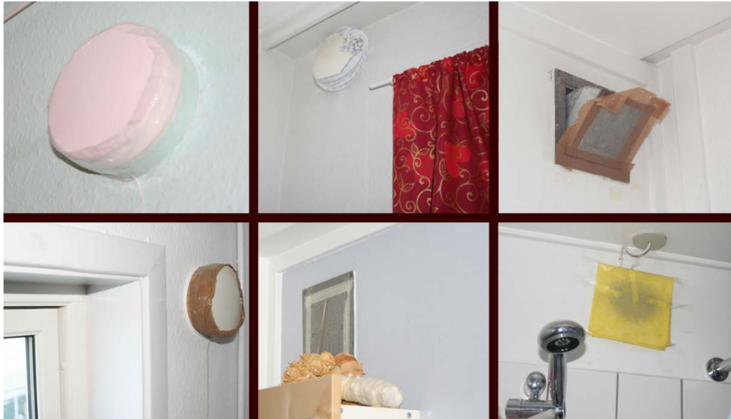
Figure 26. Sealing of the fresh air inlet to avoid cold draft in winter
