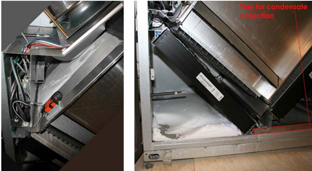
Figure 12. Frost formation in the heat exchanger and snow accumulation in the intake chamber
