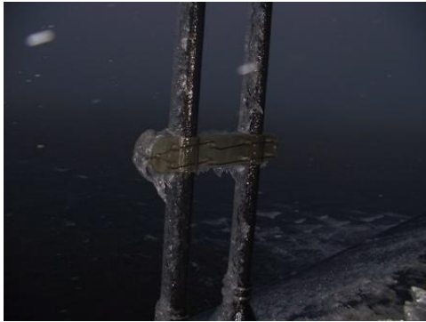
Figure 2 Iced twin hanger
