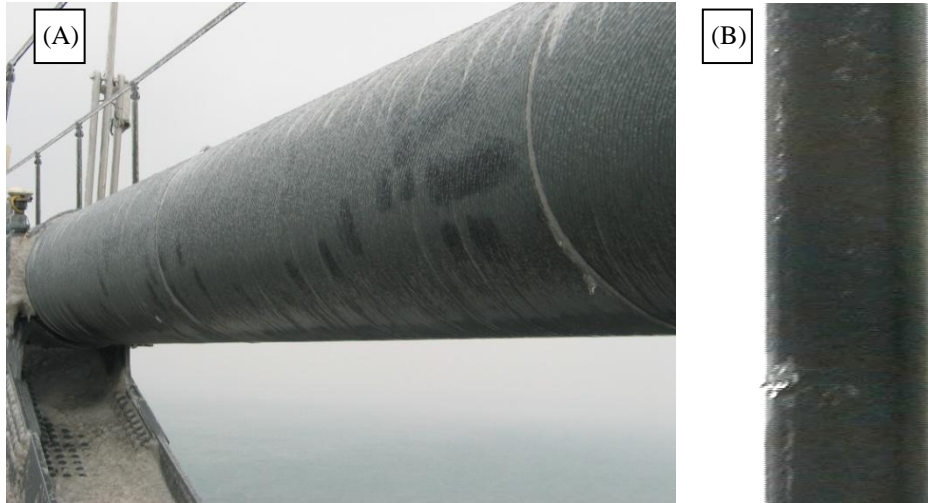
Figure 1 Iced bridge cables (A) Iced main cable, (B) Iced vertical hanger.
