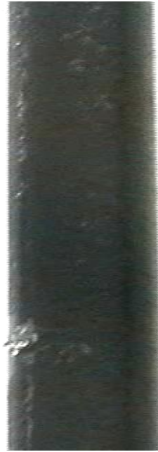
Figure 3. Iced Hanger of the Great Belt East Bridge.
