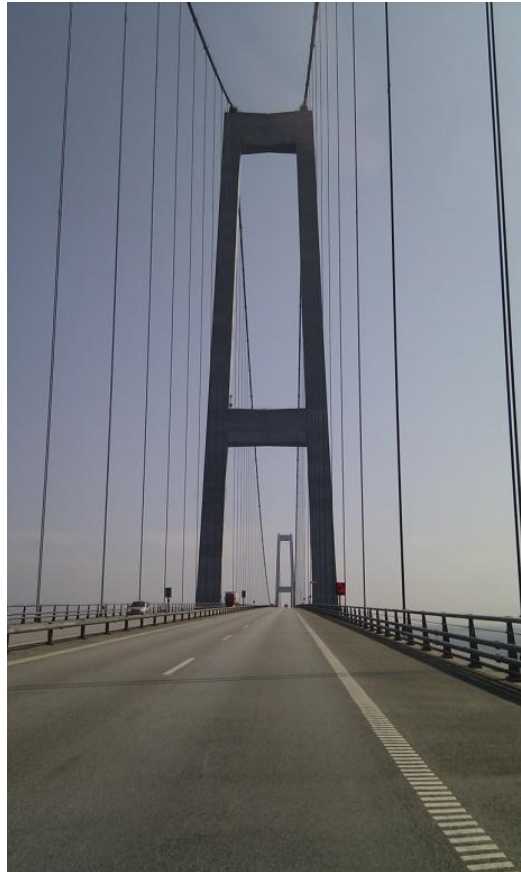
Figure 2. Hangers of the Great Belt East Bridge.
