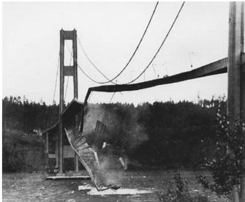
Figure 1. Tacoma Narrows Bridge collapse 1 .
