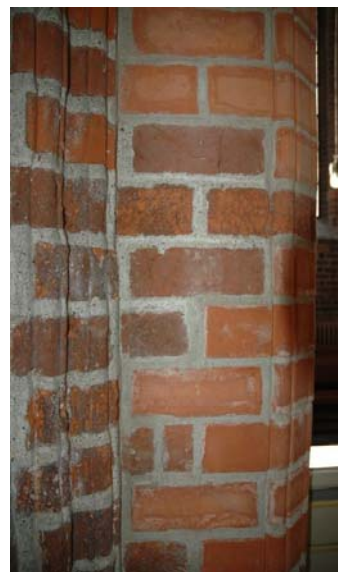
Figure 1. Picture of the pillar to the right of the altar in Sct. Mariæ Church, Helsingør, Denmark. Replacement with Falkenløwe bricks of deteriorated bricks have been carried out. Color variation is visible.
