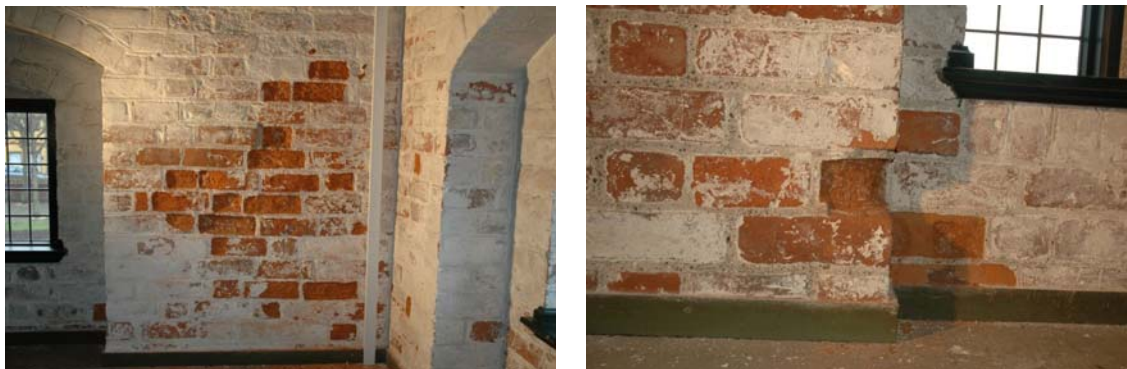
Figure 4. Deteriorated corner above the birds room. (a) Direction south-west (b) Direction north-west.
