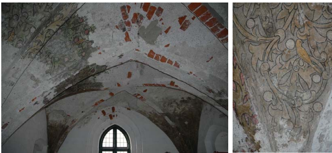
Figure 1. Extensive deterioration of the painted vault in the so-called Birds room in Vor Frue Monastery, Helsingør, Denmark. (Left) an overview (Right) a detail.
