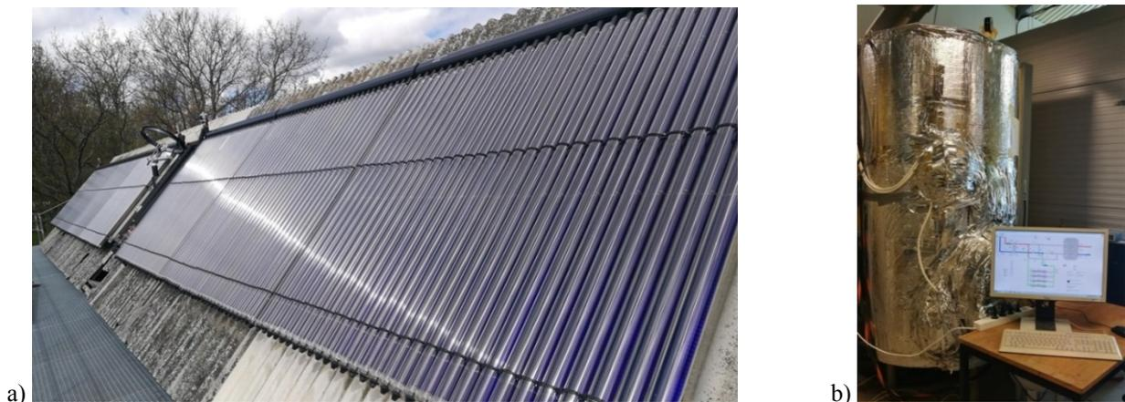
Fig. 6. a) Solar collector array; b) Water tank and graphical LabView interface for live data reading.
