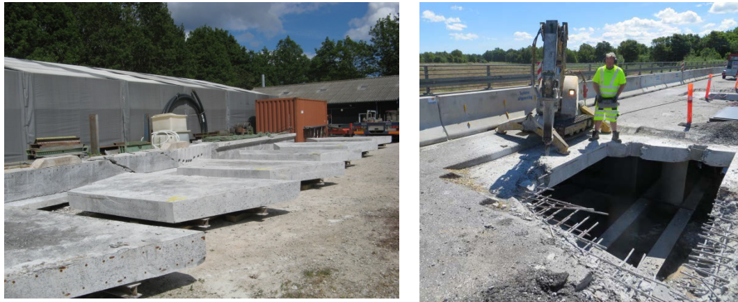
Figure 1: (a) Sawn slab segment at laboratory facility of the Technical University of Denmark. (b) The bridge slab after sawing of a segment.
