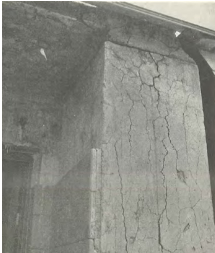
Figure 1.3: Cracking in a Danish concrete bridge. Photo adapted from (Nerenst 1952), taken in the early 1950s.
