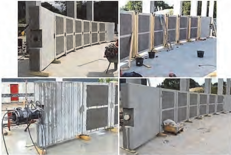
Fig. 3 Assembly steps for PC arch. 1) Top left: Vertical positioning of the elements in the desired arch shape. The dark surfaces are light aggregate concrete blocks. 2) Top right: Formwork put up and joints are cast between elements. 3) Bottom left: Two days later the formwork is removed and post-tensioning is performed. 4) Bottom right: Grouting of cable duct and the arch is ready for lifting.
