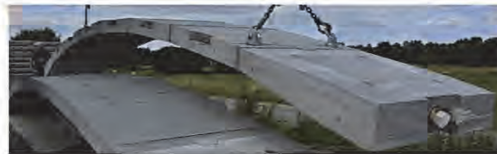
Fig. 2. Positioning of post-tensioned Pearl-Chain arch consisting of six SL Decks and two abutment elements (summer 2014). The span is 13 m.
