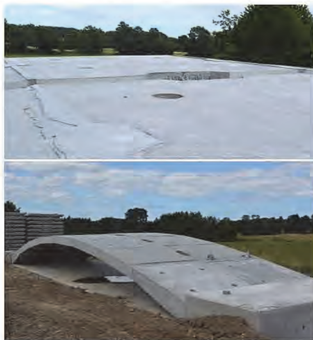
Fig. 8 Top: Close up of difference in height between the two arches at the crown showing the requirement of high accuracy during the assembly process. The first arch (closest) was placed on the foundation three weeks prior to the second arch (furthest away). Bottom: The first 13 m span PC arches in their final position.
