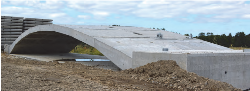
Figure 2: Two adjacent PC-Arches after assembly and lifting.
