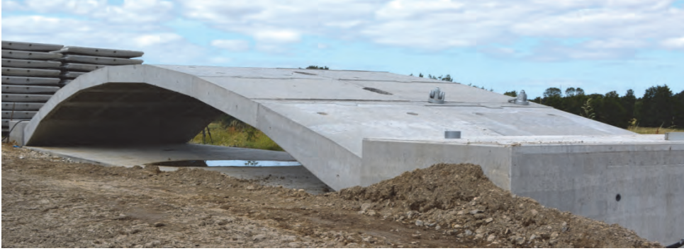
Figure 41: Two adjacent PC-Arches after assembly and lifting.
