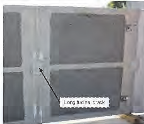
Fig. 7 Crack forming in the longitudinal direction in the bottom of the SL-deck in the joints between SL-elements. Joints between abutment elements and SL-decks did not crack due to larger number of transverse reinforcement. The dark areas are the bottom of the light aggregate concrete blocks.
