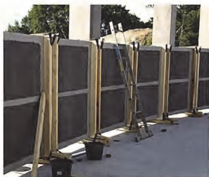
Fig. 7. SL Deck elements on edge positioned on shims on the ground during pour of joints. The bottom of the SL Decks is visible, and the darker areas are the bottom of the light aggregate concrete blocks.
