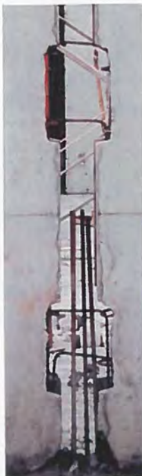
Right: Vertical internal and external open joints
