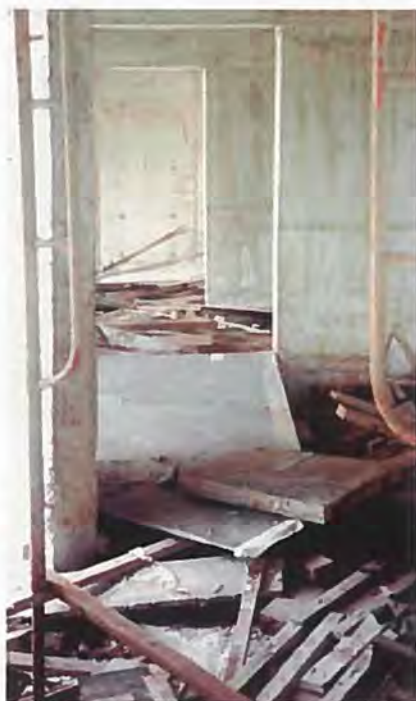
The in-situ casting construction method generates a large amount of waste, prevents access and is labour intensive both in construction, cleaning up and finishing. The PC method is clean and effective with minimum waste.
