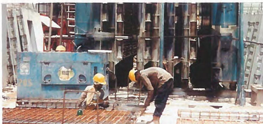
All reinforcement for battery mould castings is prefabricated and hoisted into the mould as one unit.
