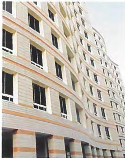
Far Right: Concrete panel cladding with cast-in granite surface
