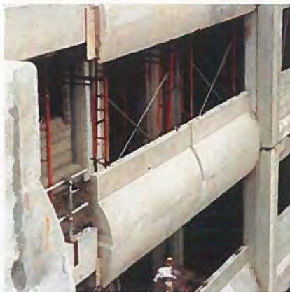
Bottom: Flexible parapet steel mould
