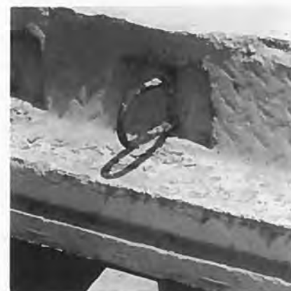
Details of mould edge, lifting hook, stirrups and cast edge with waterproofing profile.
