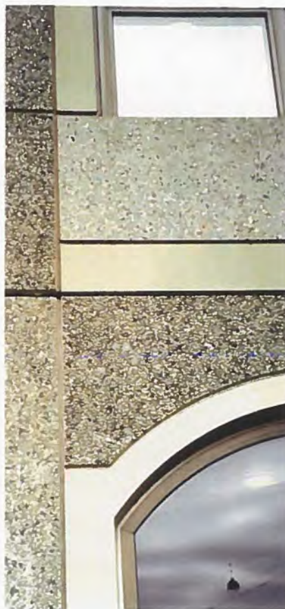
Left: Exposed green granite, fair-faced coloured concrete and polished areas - all combined on the same element.
