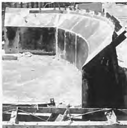
Vertical casting of complicated component
