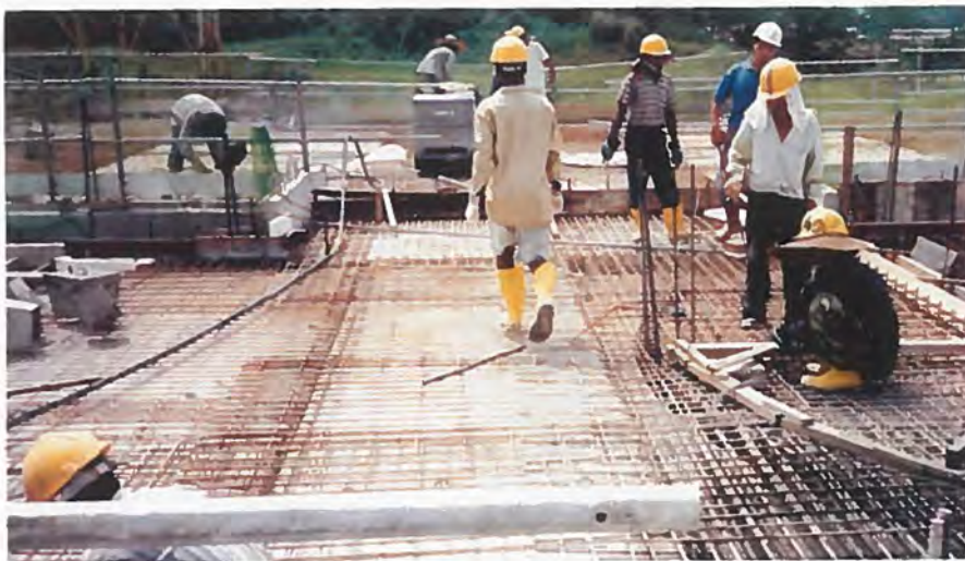
Reinforcement of topping - labour intensive process.
