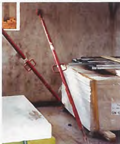
The in-situ casting construction method generates a large amount of waste, prevents access and is labour intensive both in construction, cleaning up and finishing. The PC method is clean and effective with minimum waste.
