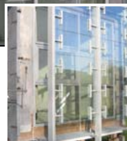
Fig. 1 The solar shading system with the lamellas in daylight redirecting position.
