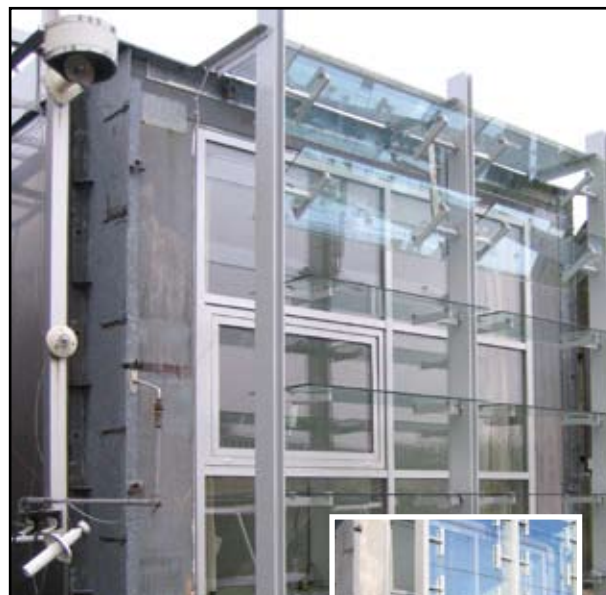
Fig. 1 The solar shading system with the lamellas in daylight redirecting position.
