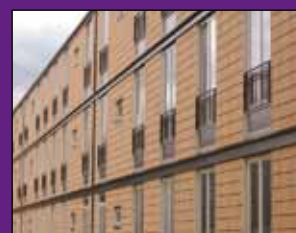
Multi-storey property after a façade renovation with an improved insulation and a new rain shield. Photo: Henrik Tommerup
