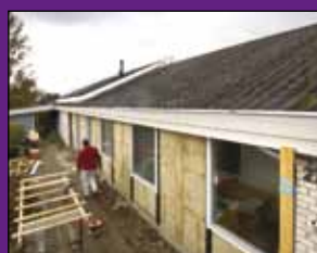
Insulation of existing exterior walls under construction in typical home from the 70's. Photo: Rockwool
